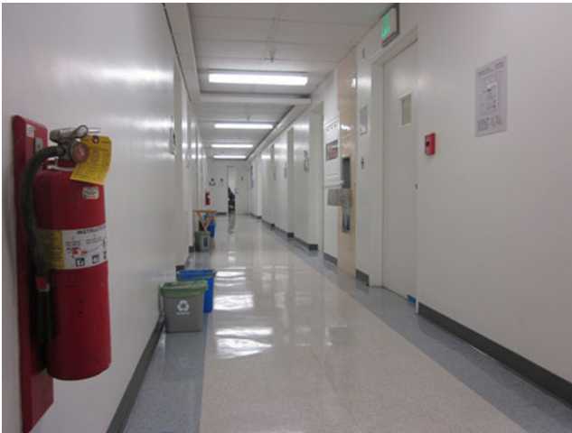
Fig. 2 A typical hallway layout in Franz Hall. The location of several fire extinguishers (two attached to wall on the left, at opposite ends of hallway; a third enclosed in a glass case on the right wall just past the water fountain, with “FIRE EXTINGUISHER” emblazoned in large red letters on the surface of the glass). Also visible are a drinking fountain (next to the encased fire extinguisher), floor plan (posted on wall, at right), and fire alarm (between floor plan and drinking fountain)
